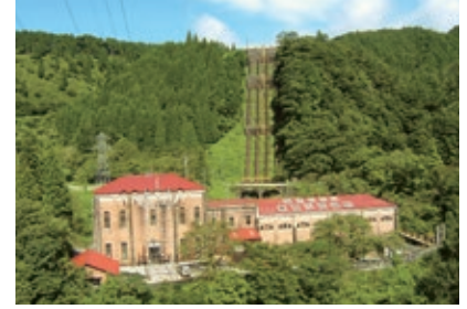
Higashi-Yokoyama power plant
