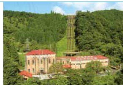
Higashi-Yokoyama power plant
