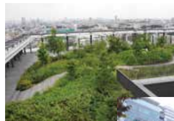
Roof greening system (Photo: NODAI Academia Center, Tokyo University of Agriculture)
