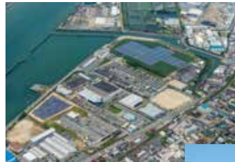
The Japan's largest water floating solar power generation
