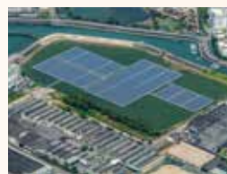
The Japan's largest water floating solar power generation
