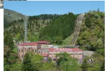
Higashi-Yokoyama Power Plant
