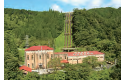
Higashi-Yokoyama power plant
